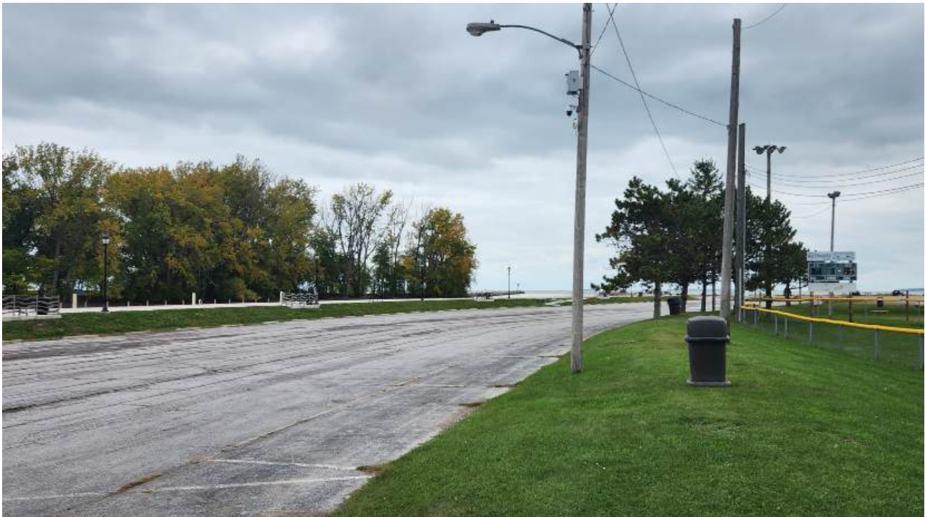
Main entrance is in need of formalization
